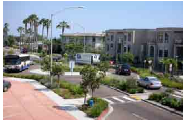
Infill/Redevelopment foreground scaled to fit in with older development background.
