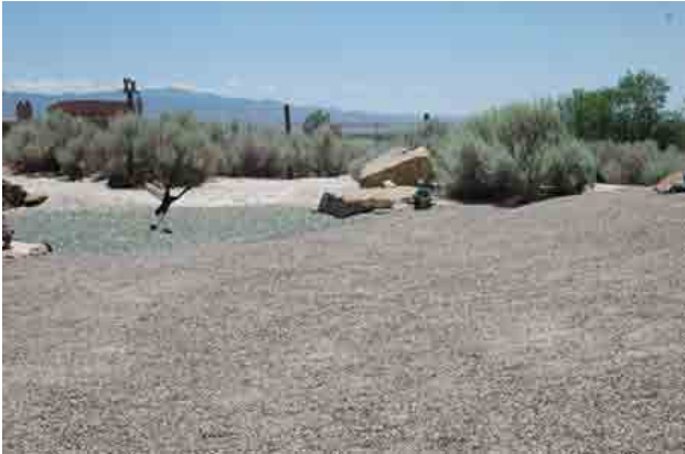
Small undulations in landscape design slows surface flow rates and reduces the risk of washout of soil downstream.
